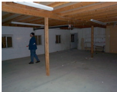
(l.) The view looking southeast towards the "Red Barn," a new facility that will offer artists the opportunity to produce work in the unique environment of the Amargosa Valley. (below) Interior of the main room of the Red Barn.
